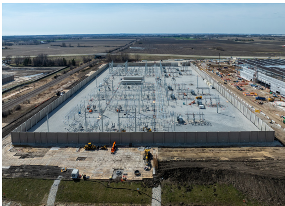
Crews construct the concrete foundation and structural frame of a large data centre facility.
