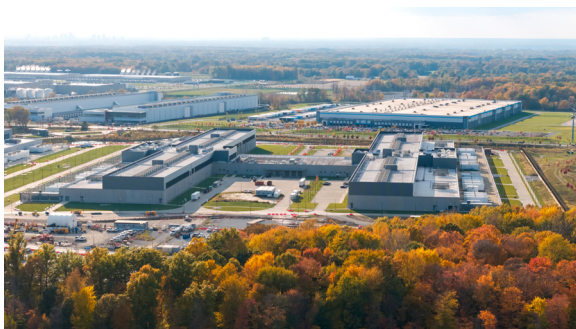
A large-scale data centre campus comprises multiple facilities and supporting infrastructure.
