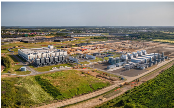
Aerial view of a hyperscale data centre campus with supporting power and cooling infrastructure.
