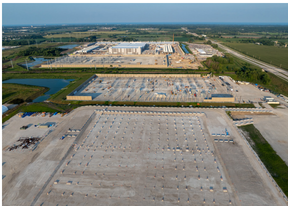
Multiple phases of construction take place across an expansive data centre campus.
